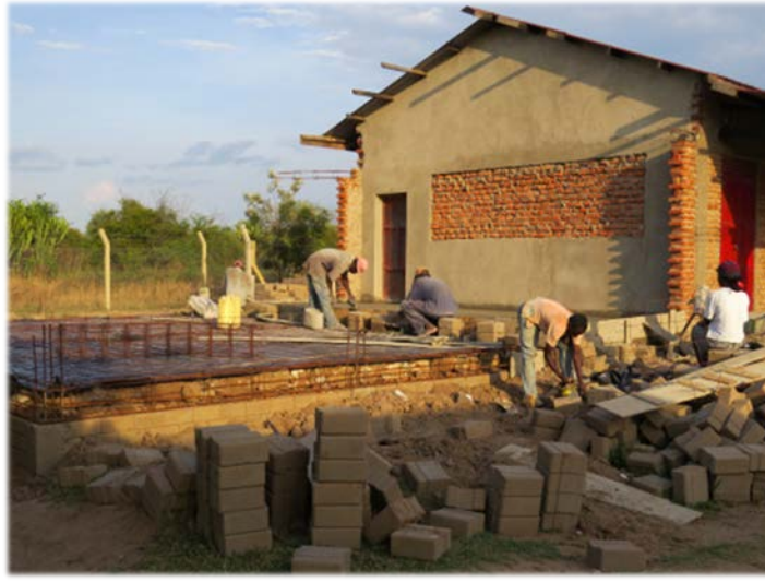
Our builders are currently working on the lunch shelter
